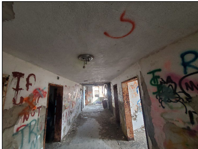
Photo 7: View of acoustical surfacing material.
