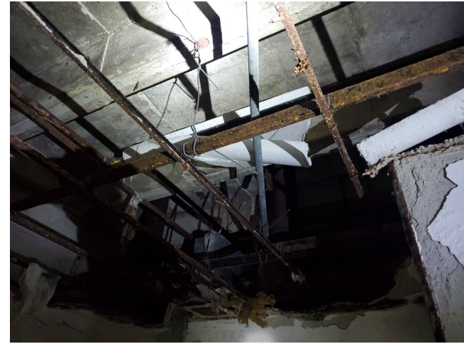
Photo 10: Mag insulation on pipe runs.
