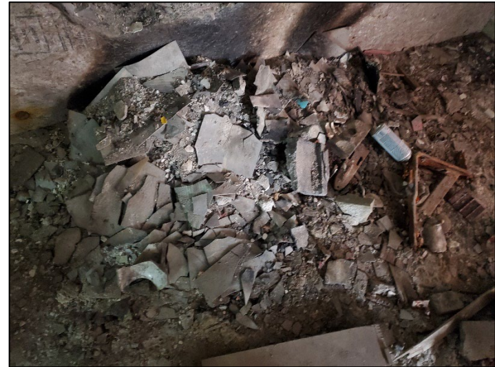
Photo 6: View of asbestos contaminated debris (typ.).
