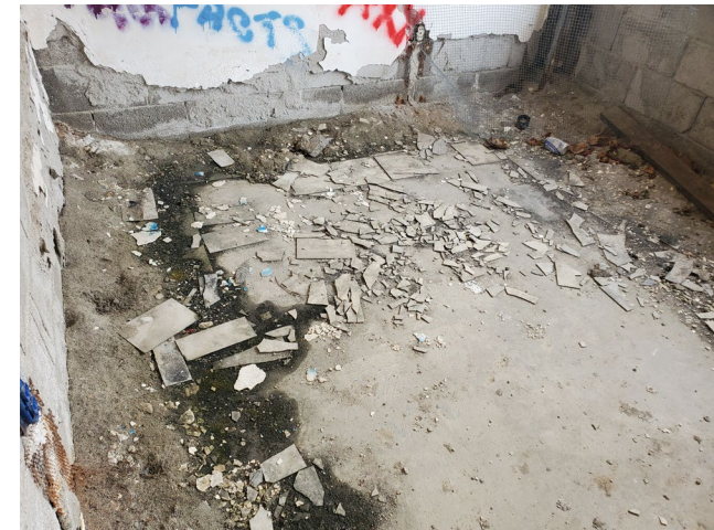
Photo 12: View of friable vinyl floor tile.
