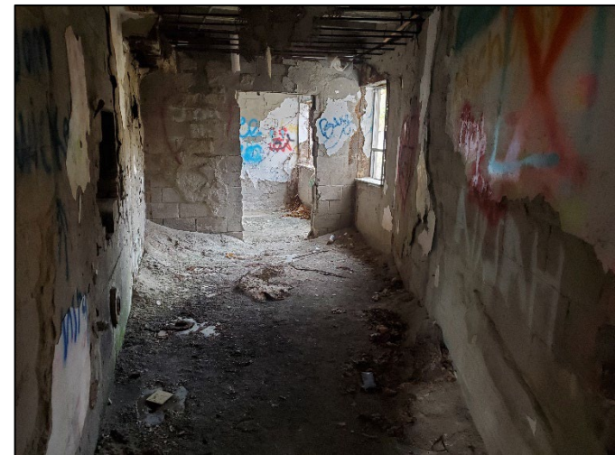
Photo 6: View of asbestos contaminated debris (typ.).
