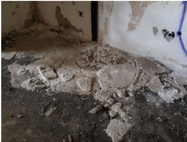
Photo 11: View of asbestos contaminated debris (typ.).
