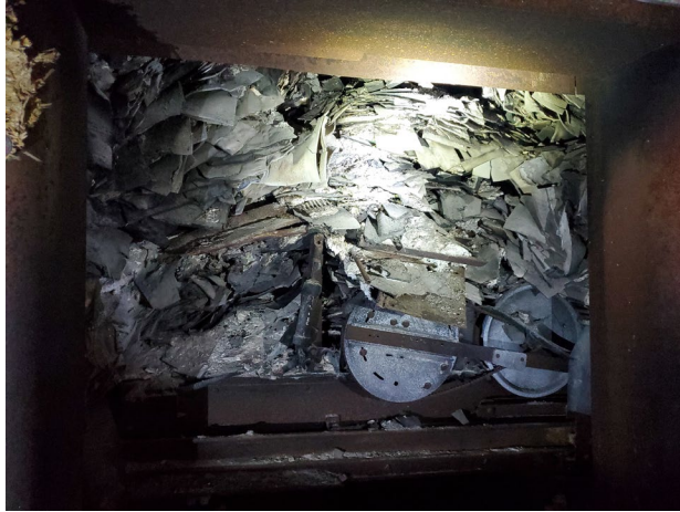
Photo 9: View of asbestos contaminated debris in the elevator shaft.
