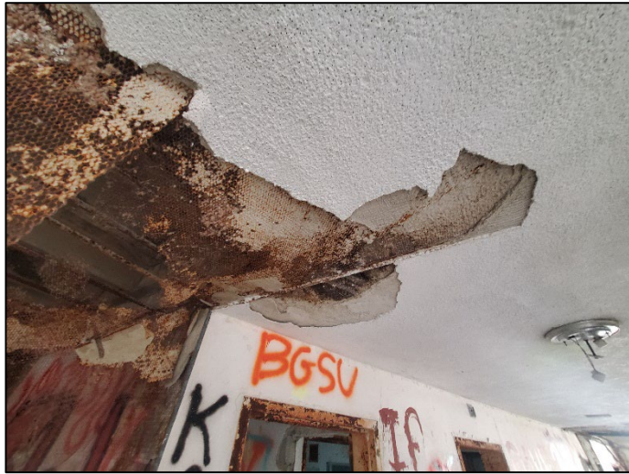
Photo 5: View of acoustical surfacing material.
