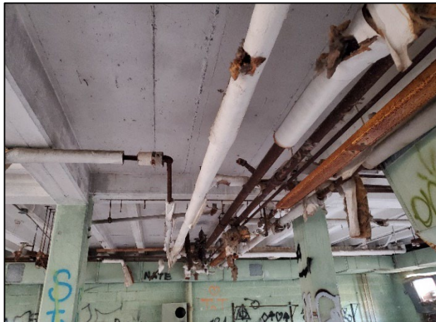
Photo 3: View of a combination of fiberglass insulated pipe, corrugated air cell, and mudded fittings.
